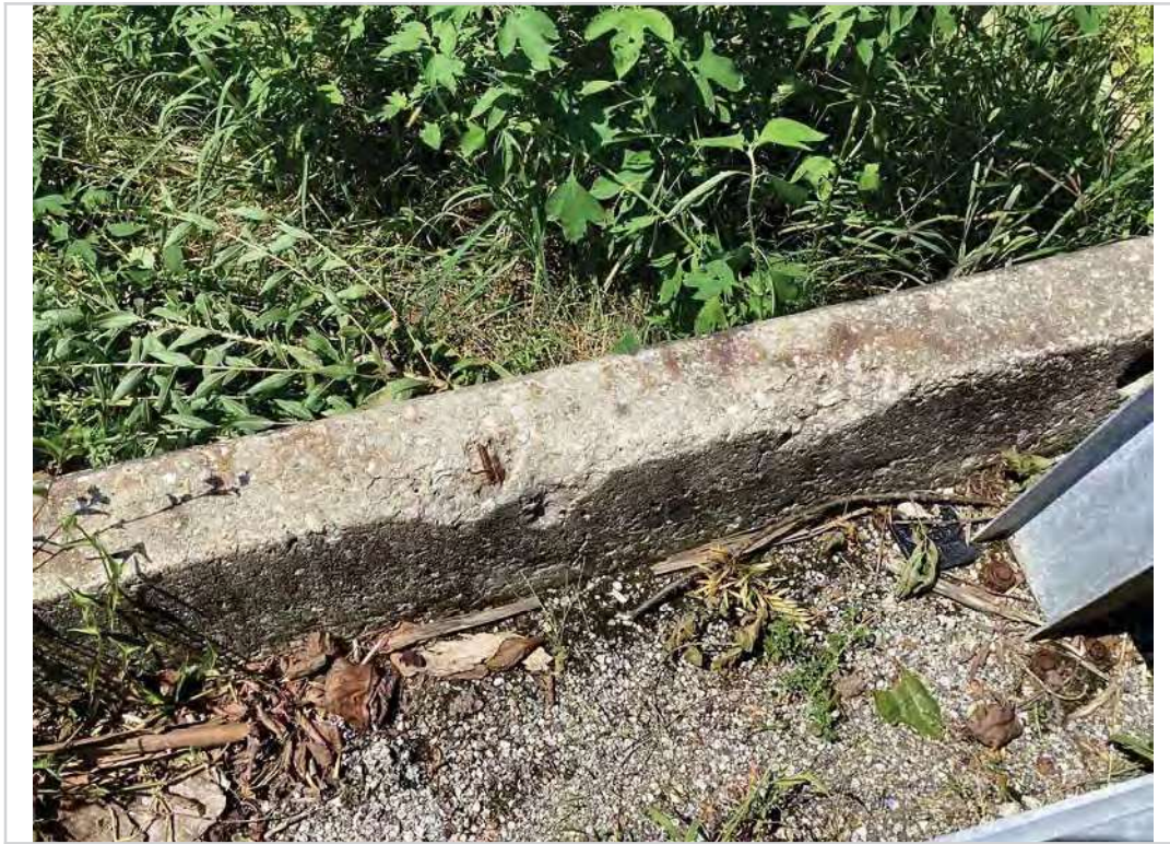
Spall to steel on left curb of span #1
