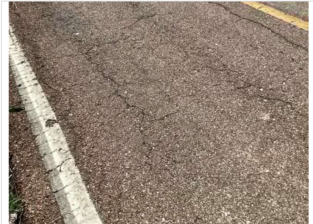
1/16" cracks on span #3 deck
