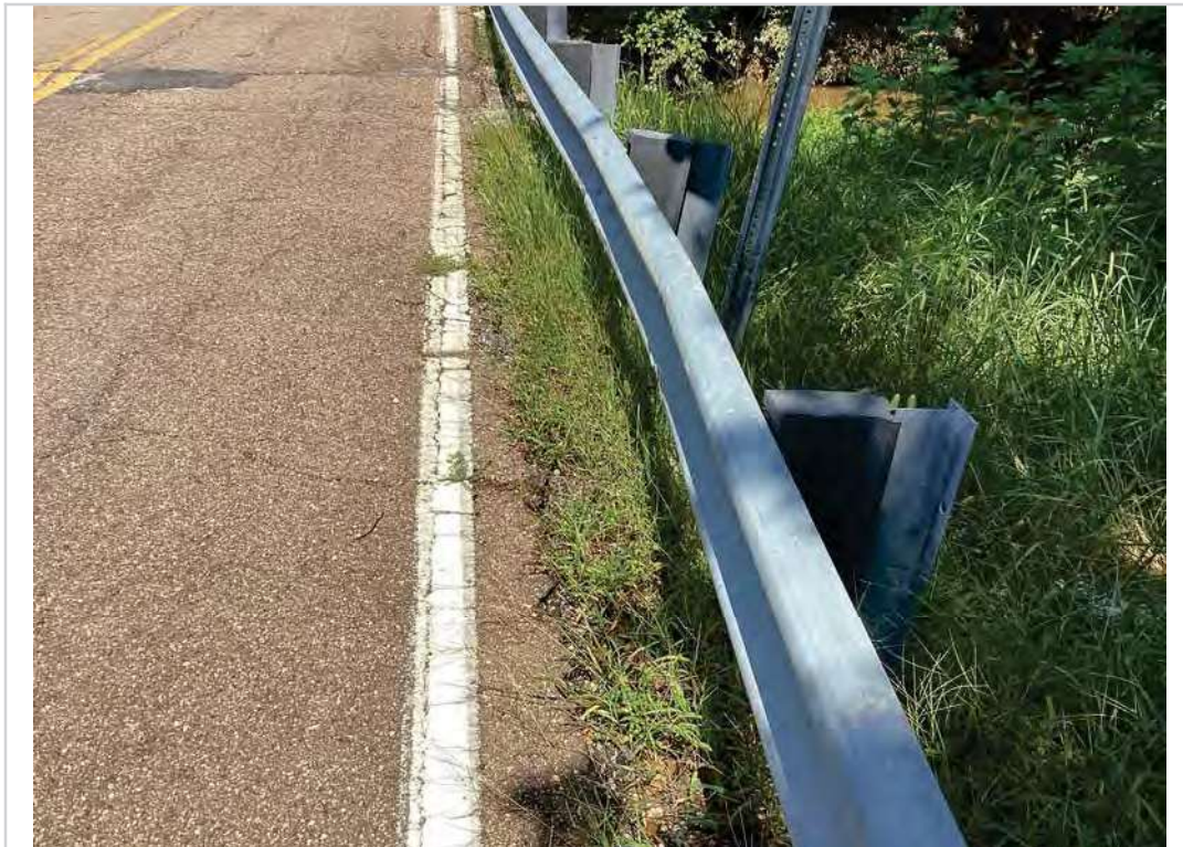
Approach 2 left guardrail damage
