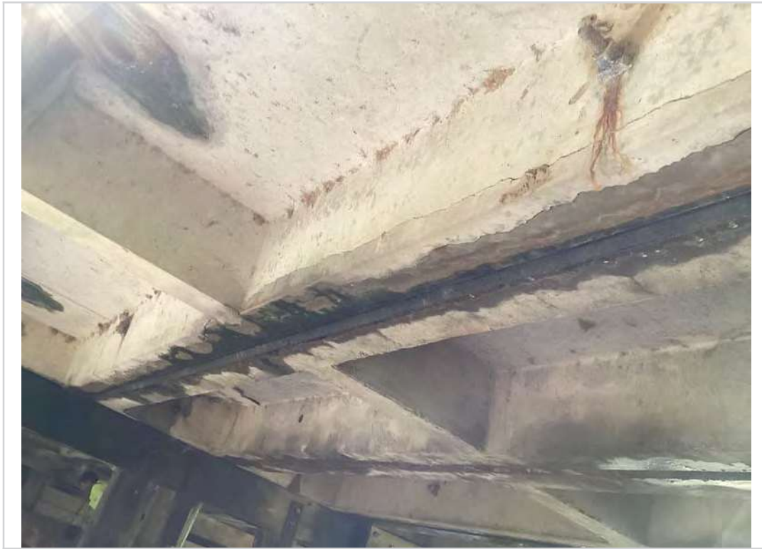
Span 2 Pre Cast Concrete Slab A impending Spall
