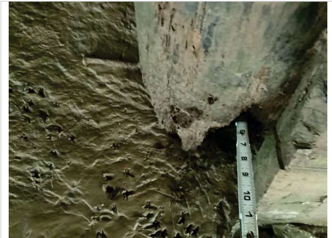
Abutment 2 pile B decay
