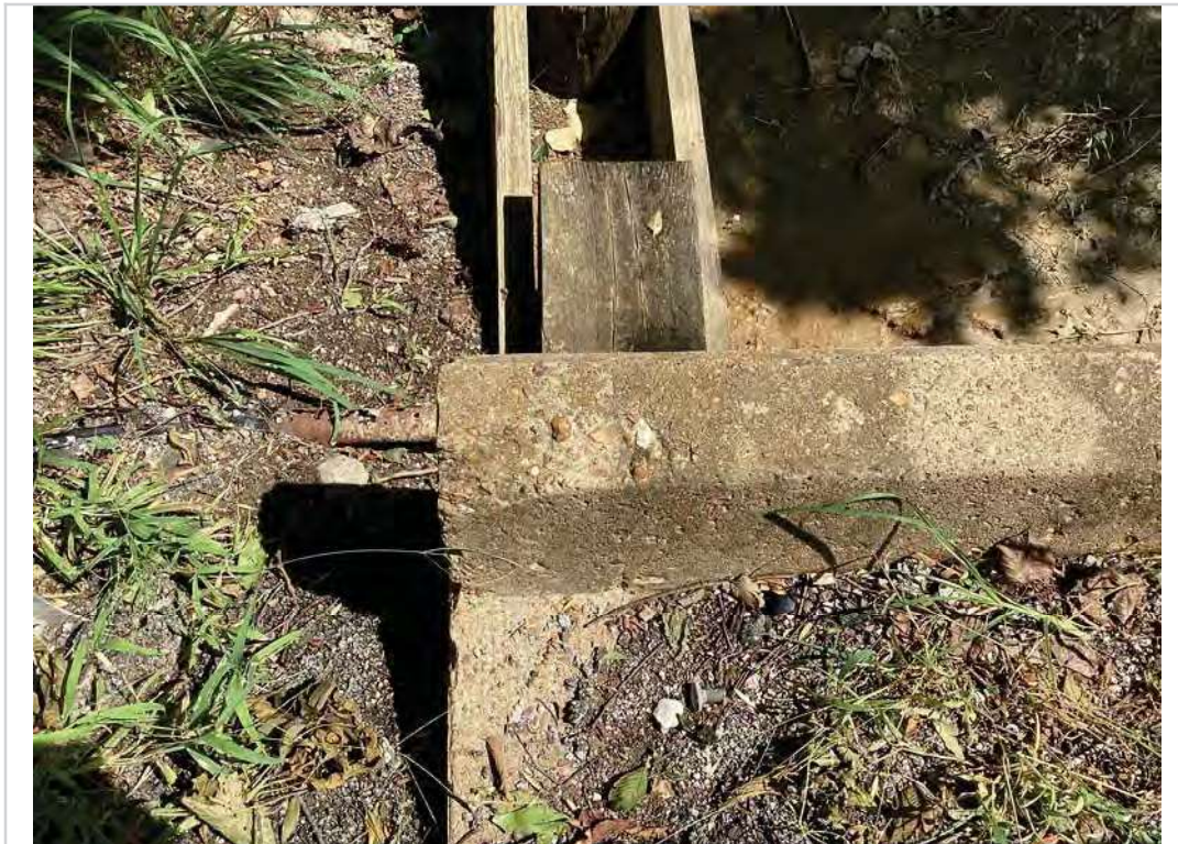
Spalling on left curb of span #1
