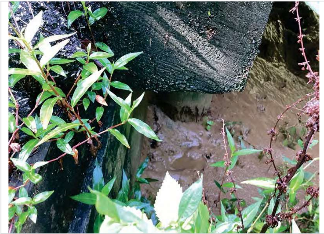
Abutment 2 Pile A decay
